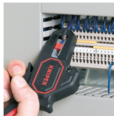
Stripping in confined areas
